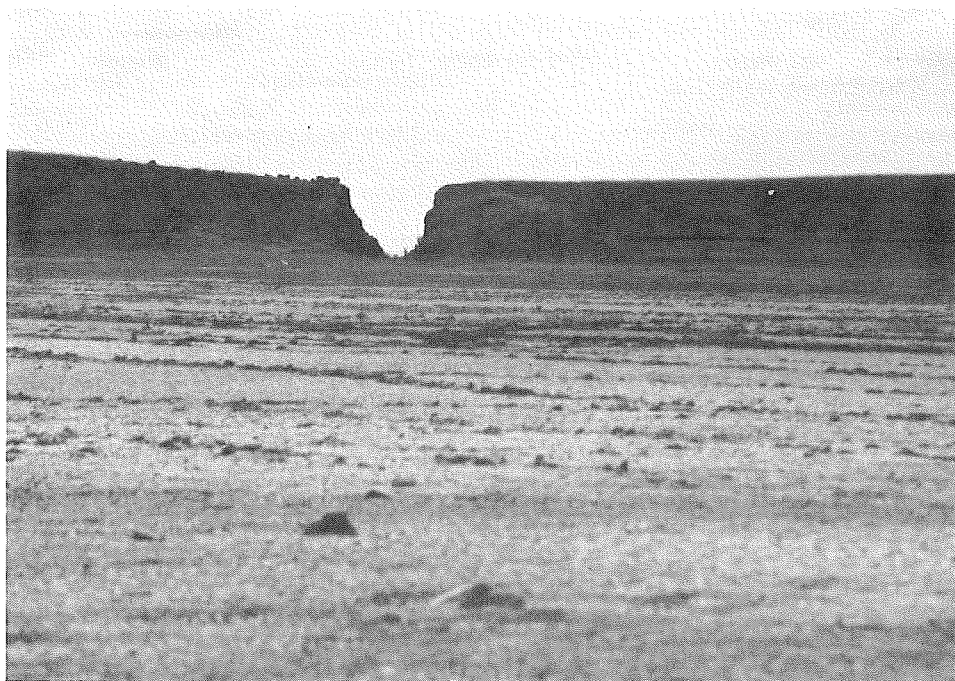
Figure 8. A cut channel through a hill on the western side of Beards Lake has drained the largest lake on the Monaro.
